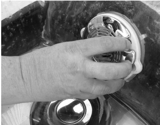
Remove screen by turning counter-clockwise.
